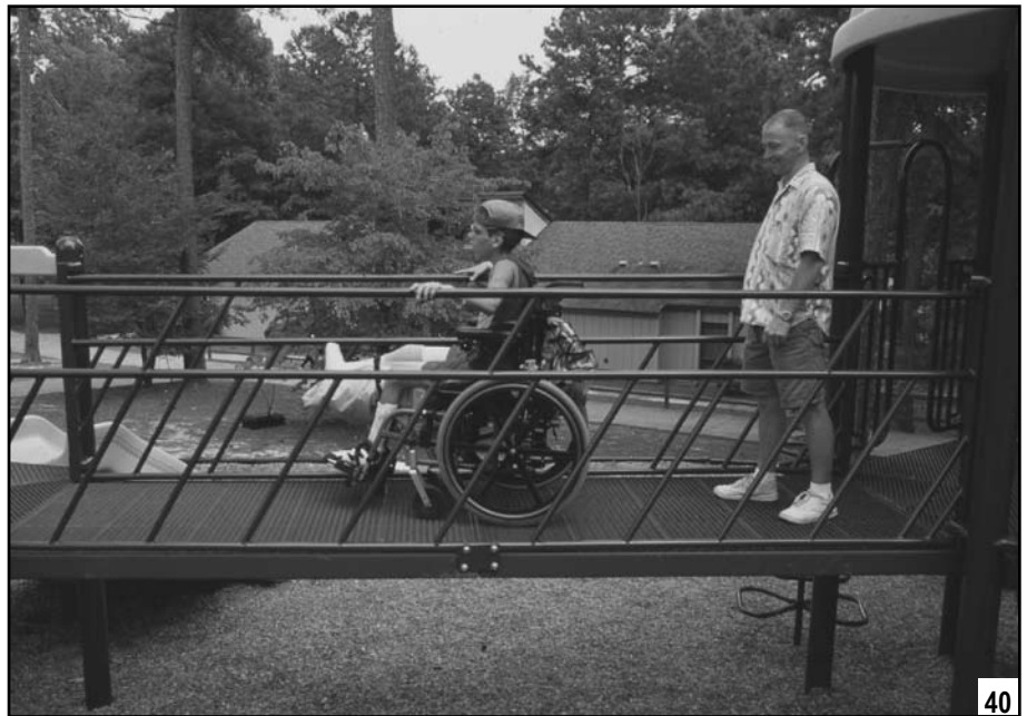
This photo illustrates an elevated accessible route:
